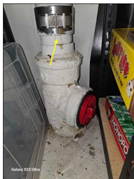
Signs of past leaks noted at the main plumbing stack.
