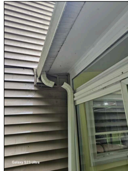
Damaged downspout extension noted front side. This should be properly sealed/repaired.
