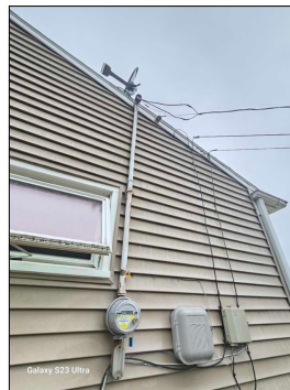
Improper drip loop noted, exterior left side
