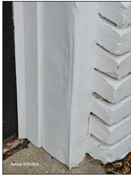
Damaged capping noted at the attached garage door frame. Monitor and repair as needed.
