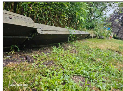
Wall failing ext rear
