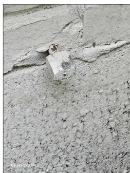
Old burp valve noted exterior front side. Not in use
