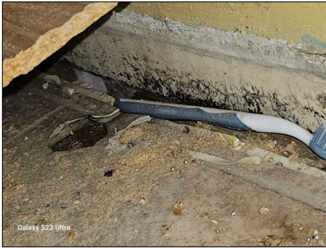
Microbial growth noted, laundry room, under utility sink
