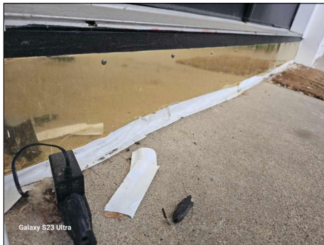
Loose flashing/ improper tape repairs noted front door. Tape is not a permanent repair and should be properly repaired.
