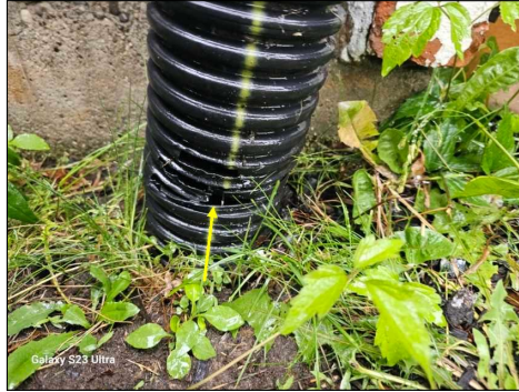
Damaged downspout extension noted front side. This should be properly sealed/repaired.
