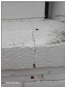
Cracked crown noted
