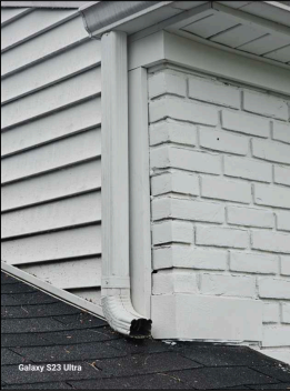
Extensions needed exterior upper level front side.
