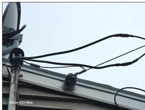
Improper drip loop noted, exterior left side
