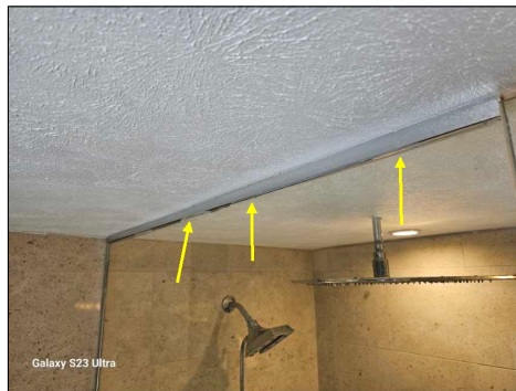
Loose pane glass noted at the master bathroom shower. This should be properly secured/repared.
